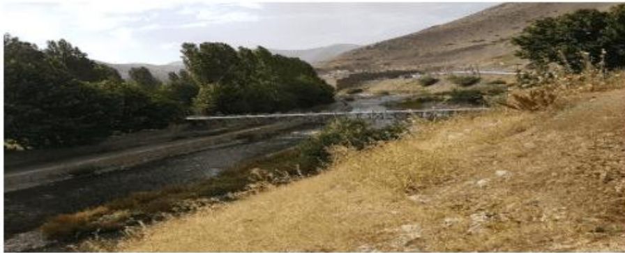
Figure 2. Existence of transverse structures on the river in interval 1
