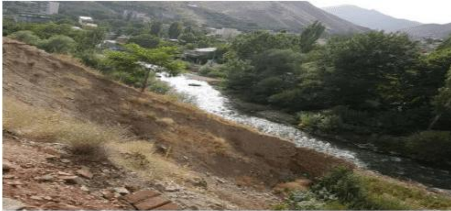
Figure 6. Existence of a steep slope along the river in interval 3.
