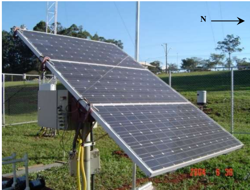
FIGURE 3 – Photovoltaic module with 100Wp each, installed in parallel, to form the photovoltaic panel of the hybrid system.
