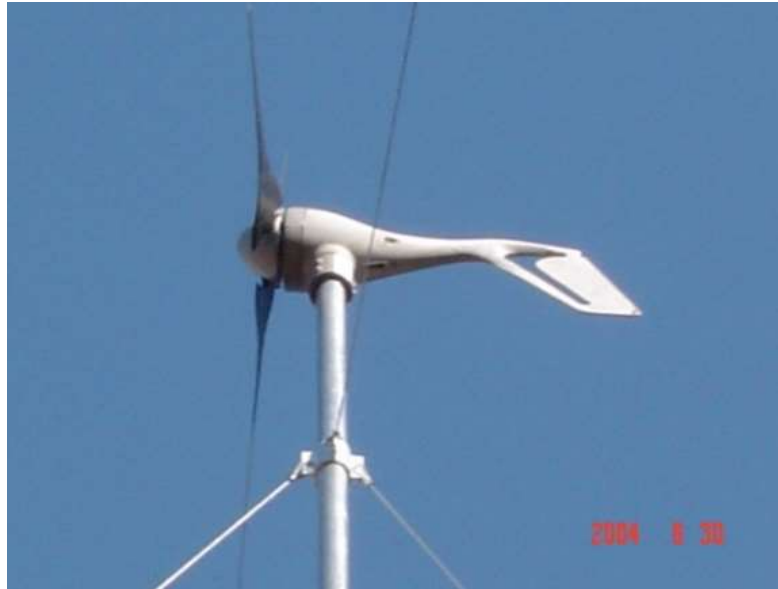
FIGURE 2 – Aerogenerator AIR-X with a 400W nominal potential installed in a hybrid system.
